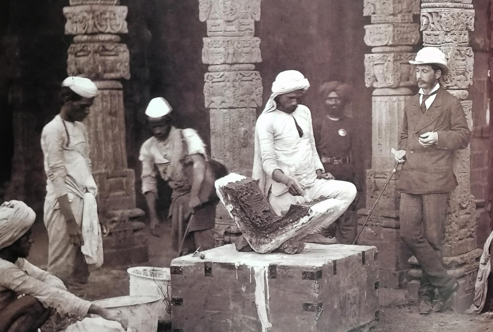
Casting operation in the courtyard of the Quwwat Al-Islam Mosque, Delhi; photography by Charles Shepherd, 1870 (source: Arundel Society. London)
